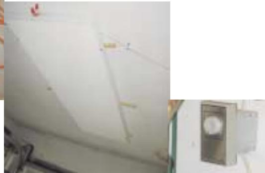
Six 24" x 72" infrared ceiling panels. Although made for a lay-in type of hung ceiling, I have had them mounted on a plaster ceiling, simply screwing them into the ceiling. They are very light, but generate a lot of direct heat. Complete with thermostat. They require 220V.
