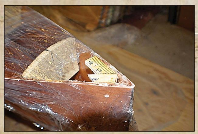
The shape of the hull and forms for the deck imposed significant bends and twists to the strips. The scrap wood (False Sheer Clamp) provided a temporary, stronger area to tack the strips until the deck was glued.
